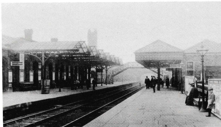
This view of the station looks towards Liverpool and shows the earlier lower platforms before electrification. The raised causeway of ballast across the tracks in the foreground was typical of most stations. Note the stone flag covering the point rodding. In the bay stands the railmotor trailer carriage, not needed today. The cutting in the distance was the scene of the crash on 25th November 1910 when 'Highflyer' No. 702 with a non-stop express collided with a stationary 2-4-2 tank standing on the wrong line. A railmotor travelling carriage-first from Maghull then ran into the wreckage in the misty darkness. The accident could not have happened in a worse place than that constricted cutting.
