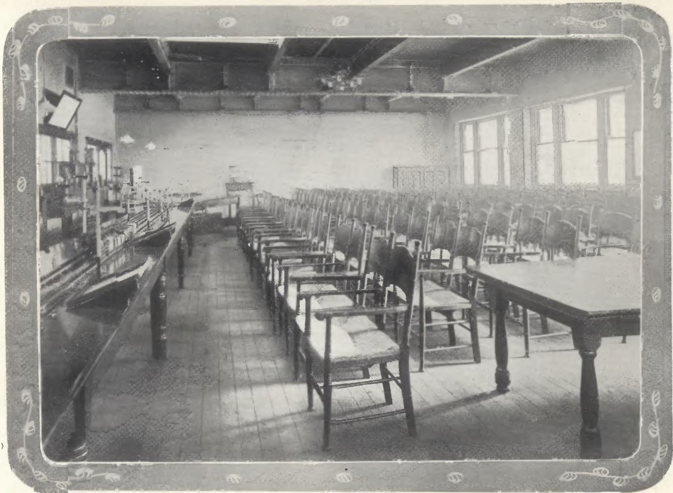
School of Signalling—Interior.
