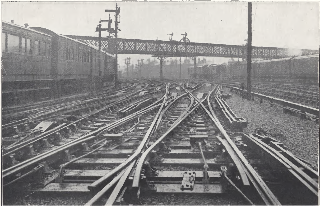
Fig. 8.—Three Sets of Double Slips at Entrance to Southport Station.
