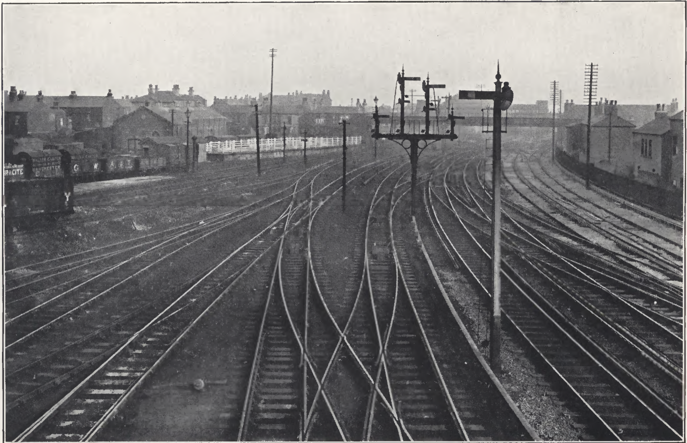
Fig. 3.—View from St. Luke's Signal Box, looking North.
