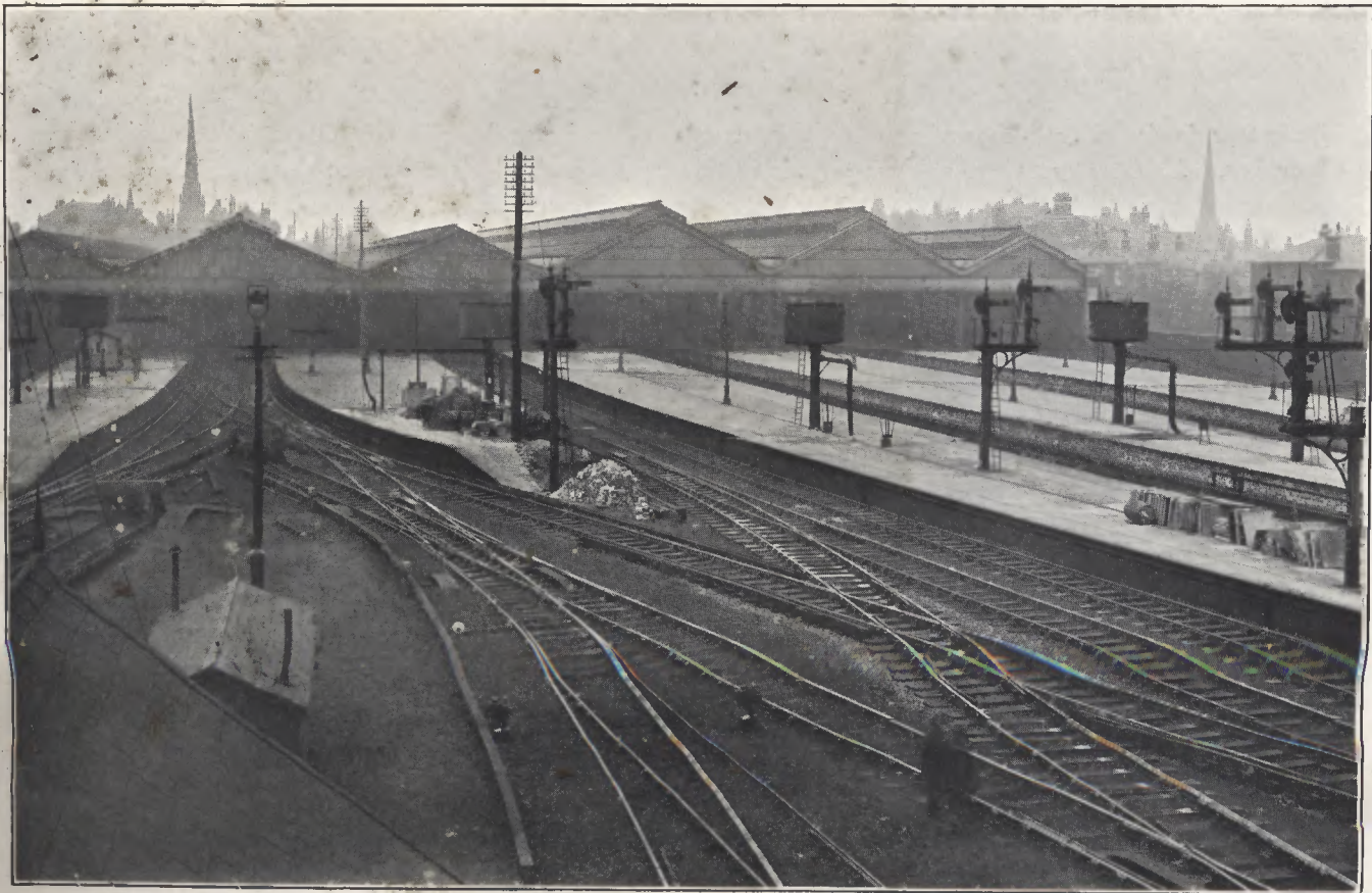
Fig. 6.—View from Southport Station Box, looking towards Station.
