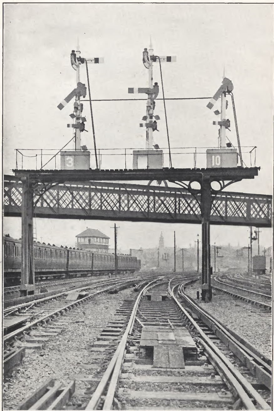
Fig. 3.—Signals with Route Indicators, Southport Station.
