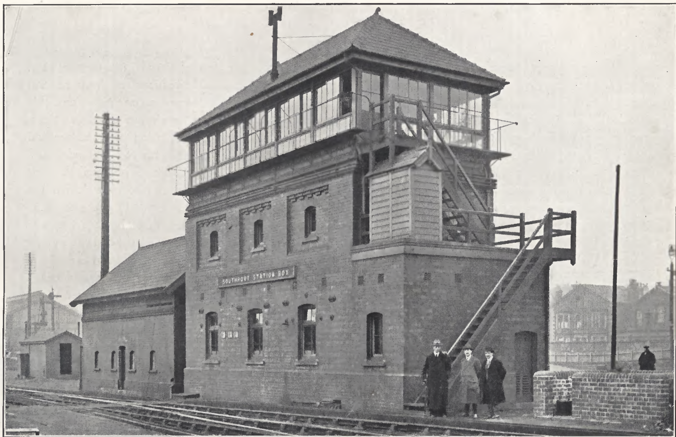
Fig. 5.—Exterior of Southport Station Box.
