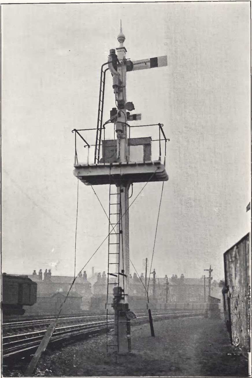
Fig. 10.—Back View of Signal No. 20 at Southport Station, with Route Indicator.
